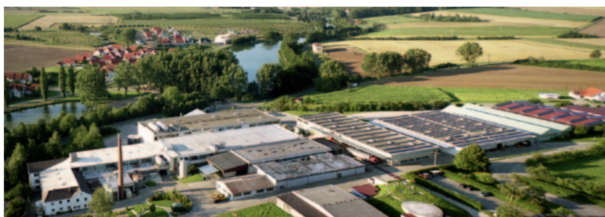
A complex structural organisation, numerous highly specialised work processes, 86,000 colour blends, in-house development work and a massive warehouse the size of two football pitches ensure that TVU is hugely successful on the global market.
